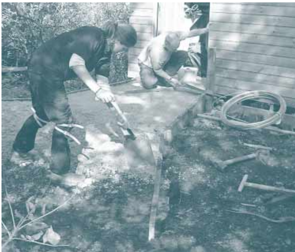
Volunteers building a wheelchair ramp at Joe's Pond
